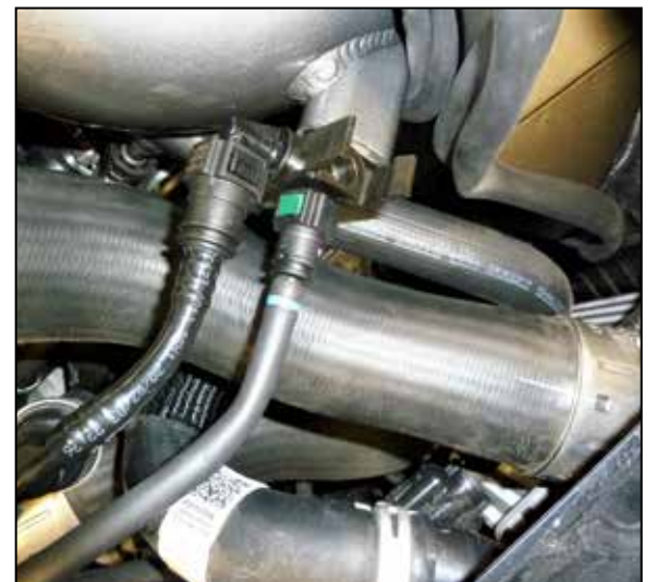
18. Reconnect the Ejector fitting vent line connections.
